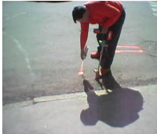
3 A Dig Safe technician applying an annotation to a road surface.
